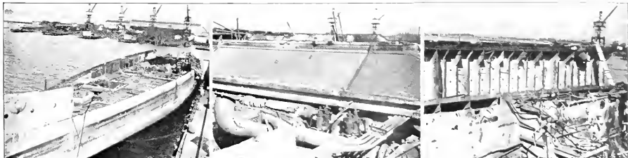
United States battleship being cut down at the plant of the Union Construction Company, Oakland, California.
